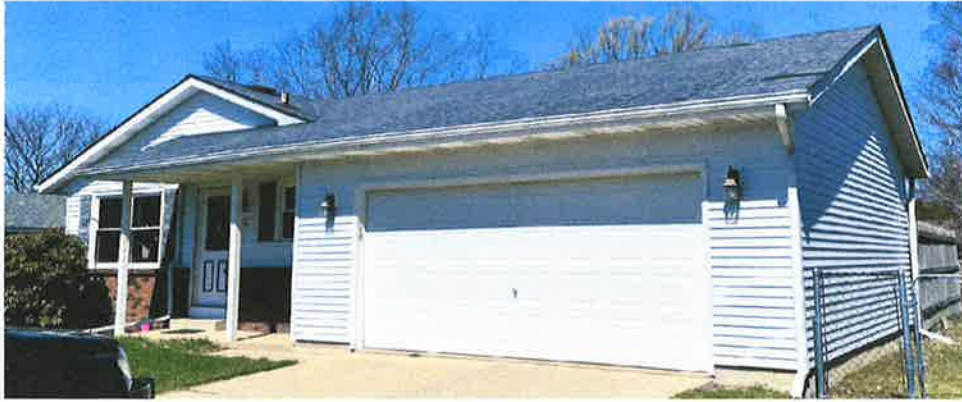
Front view from sidewalk. Sagging roof over porch, missing shingles, rusty vents, cracked garage door. Roof leaks.
