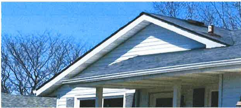
Front view from sidewalk. Sagging roof over porch, missing shingles, rusty vents, cracked garage door. Roof leaks.
